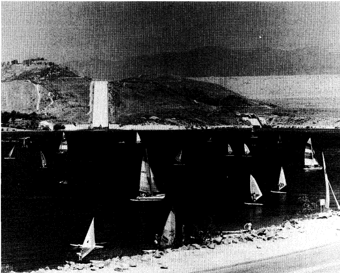
Castaic Lagoon, a facility of the SWP, is a popular recreation area for Southern California residents.
