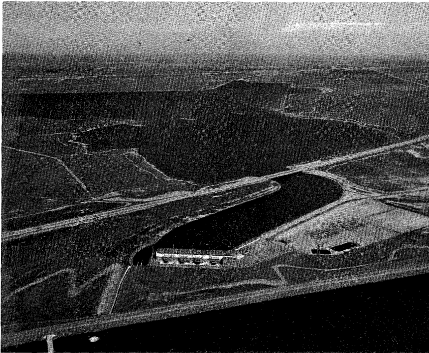
O'Neill Forebay with San Luis Pumping Generating Plant in the foreground. The Forebay is used in conjunction with San Luis Reservoir to regulate water by the SWP and the federal CVP.
