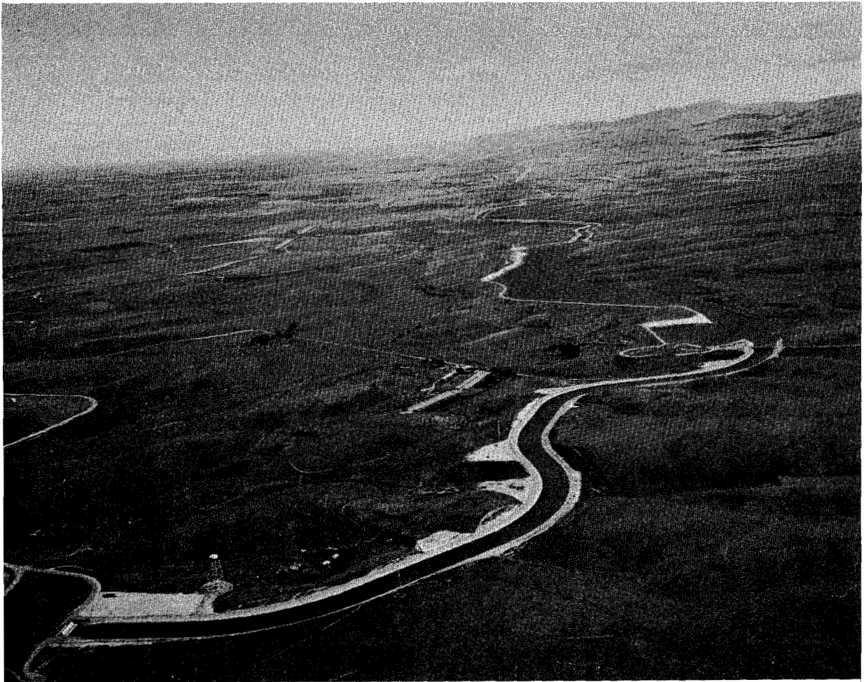
Looking southerly from the start of the California Aqueduct (shown in the lower left hand corner of the picture). The aqueduct extends to Bethany Reservoir then continues southerly through the San Joaquin Valley to Southern California.
