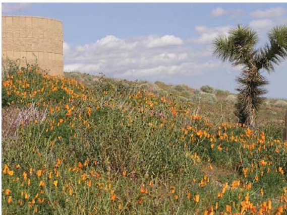
Water storage capabilities, such as tanks, are a key asset in a region where valuable water is lost daily due to a lack of available infrastructure.
