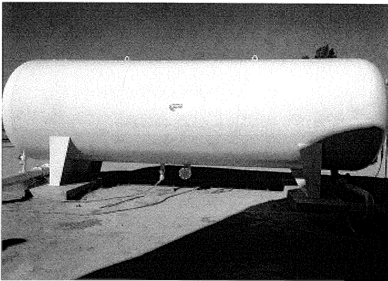
ZONE A 10,000 GAL STORAGE TANK
