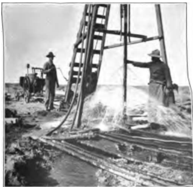
B. INSERTING PERFORATED CASING IN PARTLY COMPLETED ARTESIAN WELL.
