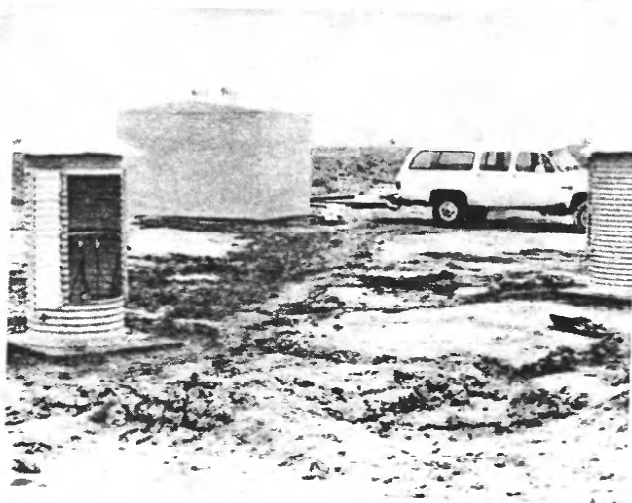
Figure 9. Holly extensometer site, looking east. Extensometer is in large building in center. Observation wells are in small, round buildings. Land-surface elevation is 2,302 feet. Photographed August 1990.
